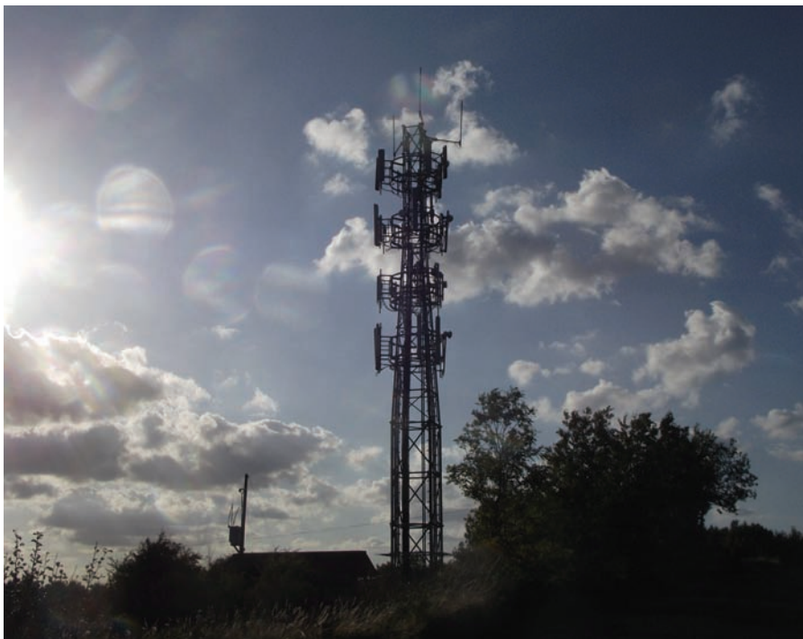
With much site sharing of towers or other infrastructure taking place across Africa, an external neutral player is taken on to run the field maintenance
