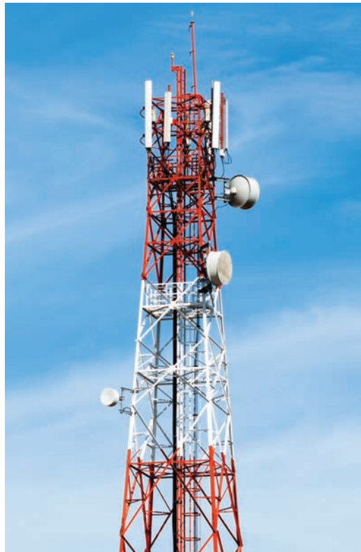
Network base stations are the nodes of any mobile system, the points of signal intersection and the points from which signalling branches out
