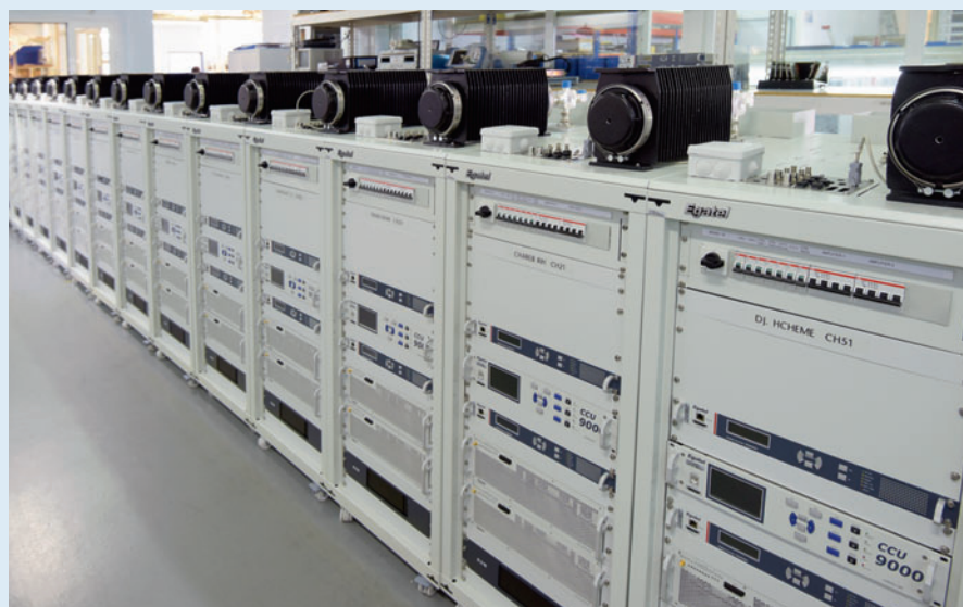
Egatel is supplying and installing equipment in Algeria for TDA
