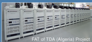
FAT of TDA (Algeria) Project
