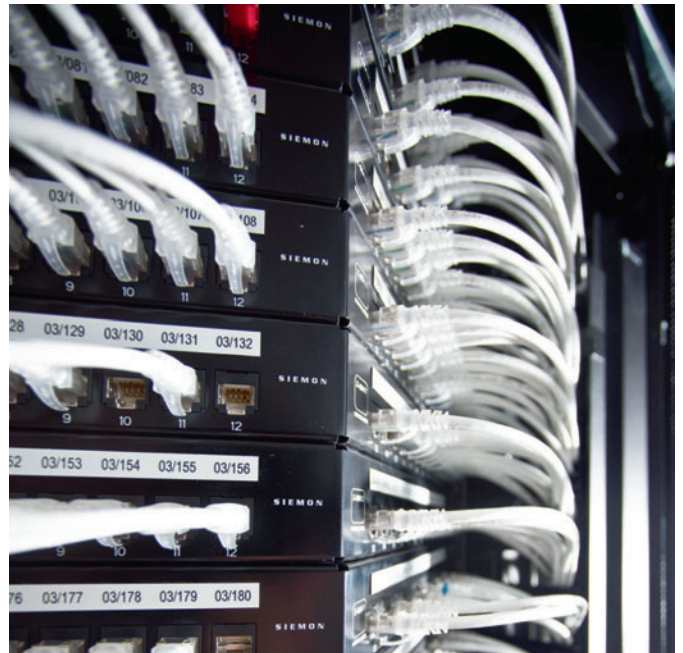
Data centre managers must select cabling media to ensure support for business growth
