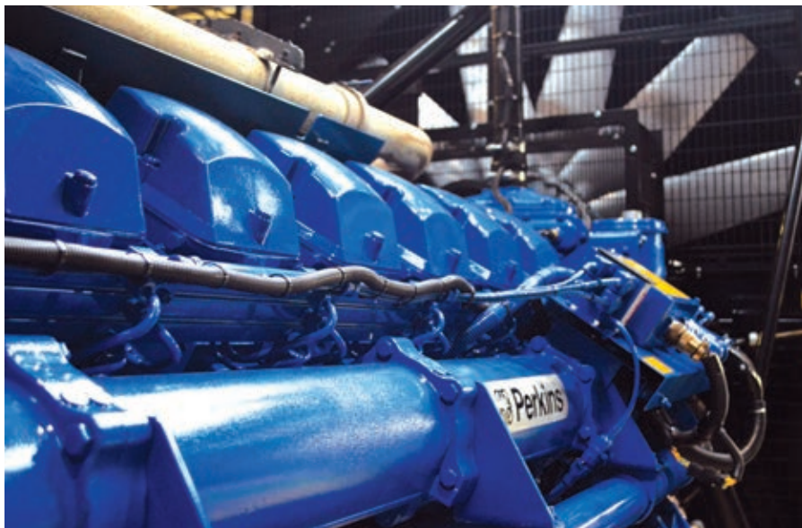
An FG Wilson Generator Set powered by a Perkins 4000 Series engine.
