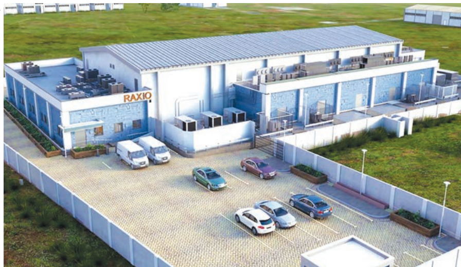
Raxio Data Centre Uganda on the outskirts of Kampala.
